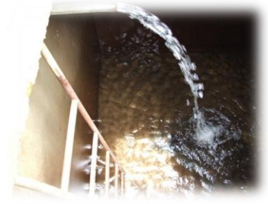
12 gpm entering the original storage tank in El Encinal
