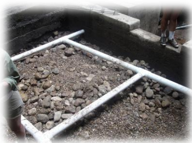
PVC filter installed at the dam site
