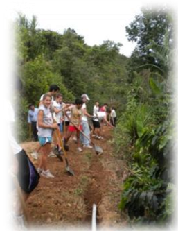
Student volunteers burying recently installed PVC pipe
