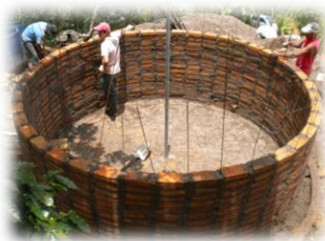
Construction of the new storage tank
