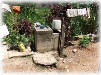
Typical pila (water storage unit) in a home in El Encinal
