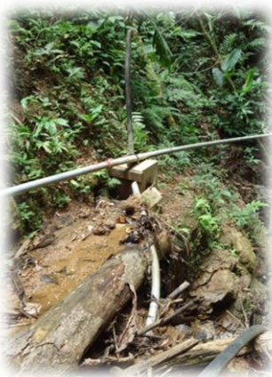
A cement anchor stabilizes the new piping in the conduction line donated by FORCUENCAS. The former piping installed by Water Brigades was bent by the force of the storm and can be seen in the lower front of the picture partially covered by debris.
