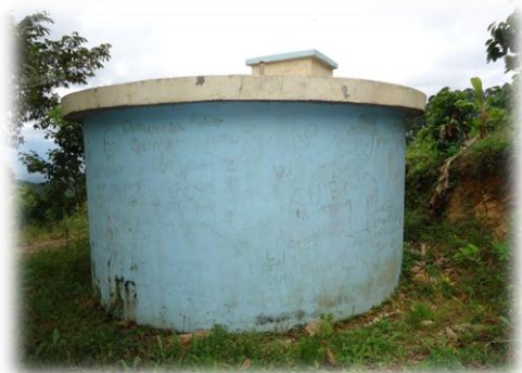
Central storage and treatment tank in El Encinal still functions well but needs a protective fence and some foundational repairs.
