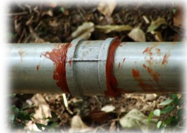
3" Galvanized iron pipe installed for the first 48 meters of conduction line
