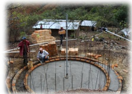
Construction of the new 5,000 gallon storage tank in Guaricayán
