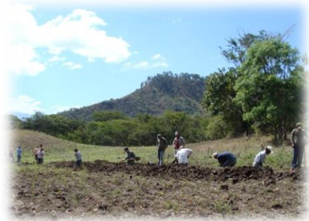
Student volunteers dig trenches with community members where they would later install piping for the new conduction line
