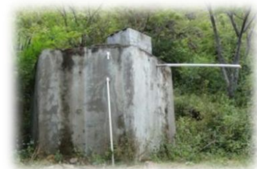
Original storage tank
