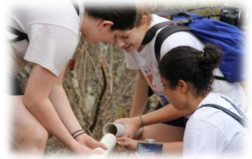
Student volunteers installing PVC piping in the distribution network
