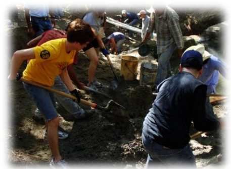
Student volunteers work with community members on construction of new dam
