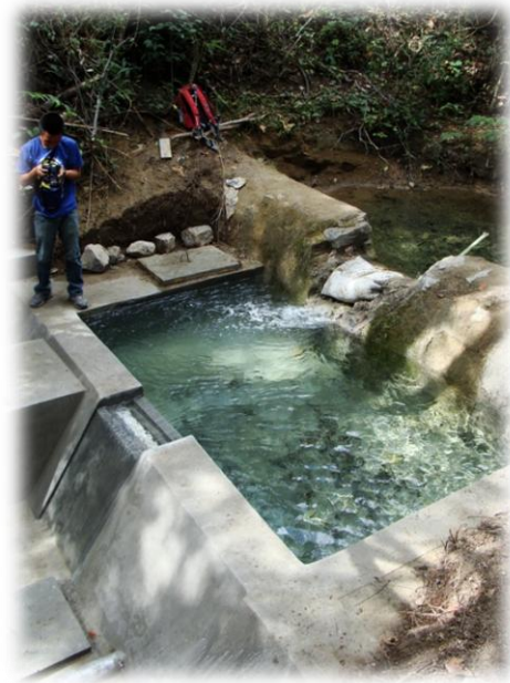
Finished and functioning dam of new system
