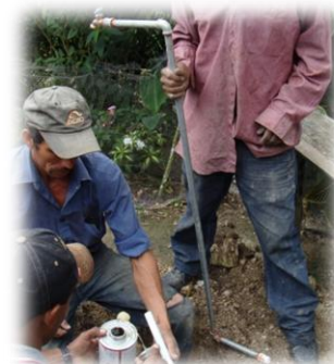
Installation of a new household connection
