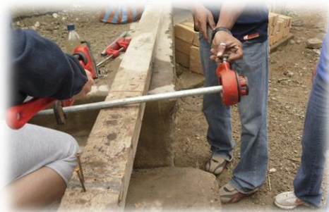
Fabrication of household connection: Pipe being threaded
