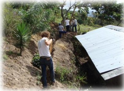
DePaul University students dig trenches for installation of new distribution network
