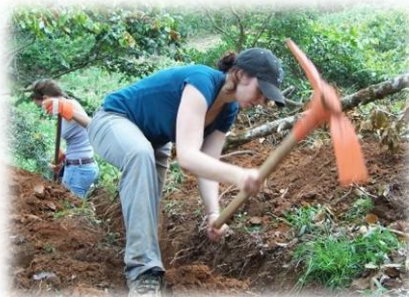
Students pickaxing trench for conduction line
