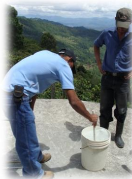
Plumber being trained on chlorination process
