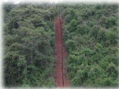
Trench dug for conduction line
