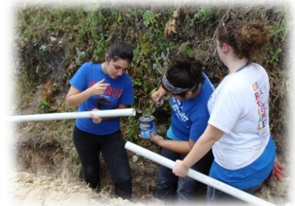
Distribution network pipes being glued together
