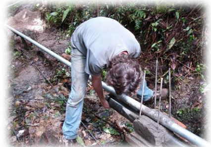
Installation of first lengths of GI pipe in the conduction line
