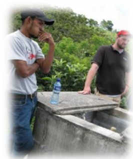
Reviewing original chlorinator
